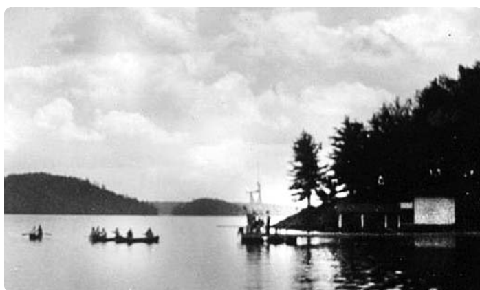
The old dock at Bona Vista
